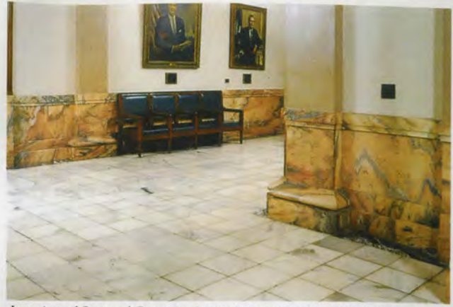
Interior of State of Georgia Capitol, Atlanta, GA. This is the original tile floor and wainscoting, installed in 1884. The floor remains in excellent condition. Georgia Marble tile is the world's best.
