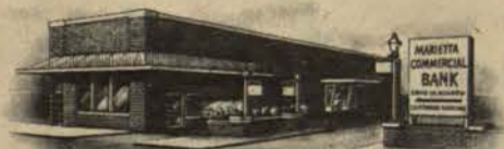
BRANCH OFFICE—114 CHURCH ST.
