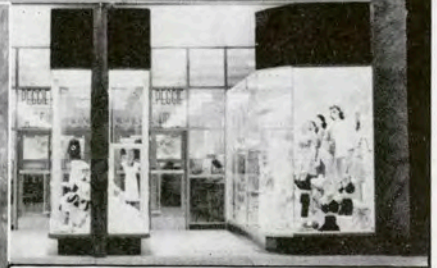
With the exception of the name panel, Etawah Pink Georgia Crystalline Marble has been used on these 23 Store Fronts. Sydney H. Morris & Associates, Chicago, Illinois, are the architects.
