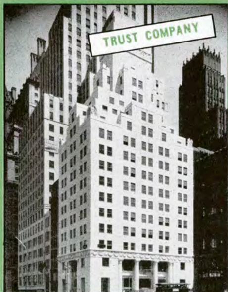
MANUFACTURER'S TRUST CO. BLDG., N. Y. C. Cross and Cross, New York City, Architects White Georgia Crystalline Marble
