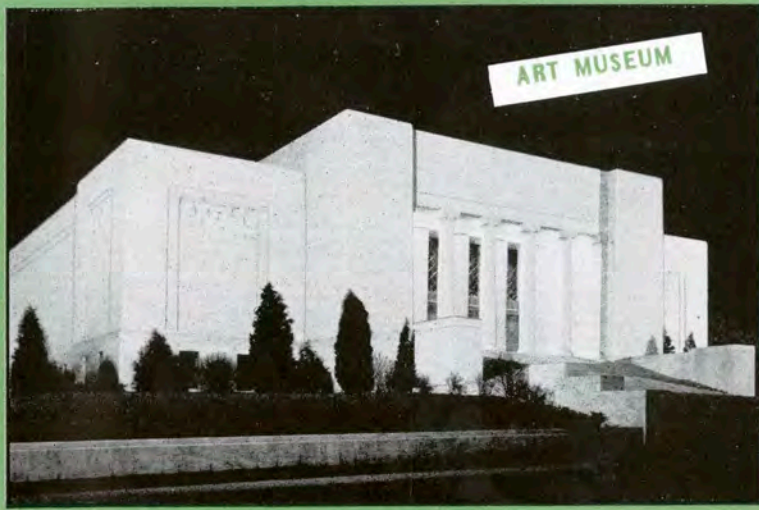
JOSLYN ART MUSEUM, OMAHA, NEB. John and Alan McDonald, Omaha, Neb., Architects Etowah Pink Georgia Crystalline Marble
