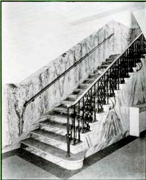
HALL COUNTY COURT HOUSE, GAINESVILLE, GA. Daniell & Beutell, Atlanta, Ga., Architects Mezzotint Georgia Crystalline Marble
