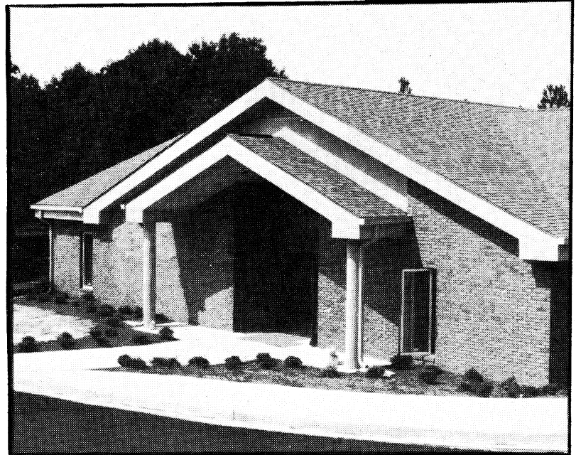
Here's the church; here's the steeple; open the doors; see all the people. Except in this case it's not a church, there is no steeple, and if you open the doors, all you see are workmen putting the finishing touches on the building. -Photo by Jack Silver
