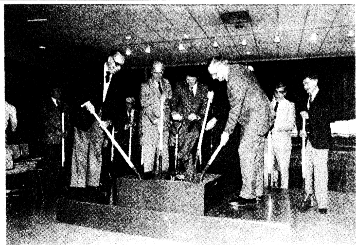
A turn of the shovel completes the indoor groundbreaking
