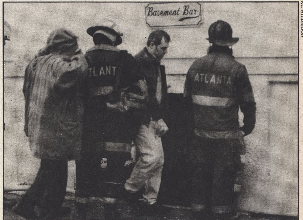
Gallus owner Don Honeywell surveys the fire damage with Atlanta firefighters.
