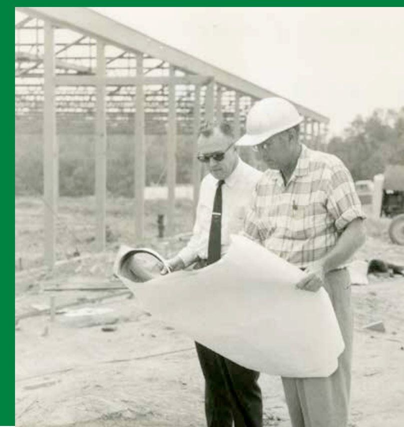
Former Southern Tech Director L.V. Johnson reviewing construction at the new Southern Tech campus in Marietta, 1961
