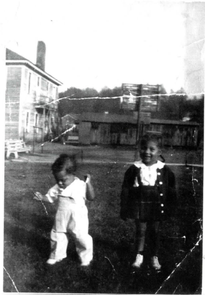
The rear of the public School Building.
