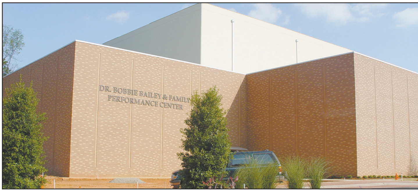
Construction on the Dr. Bobbie Bailey and Family Performance Center nears its end as the opening approaches.
