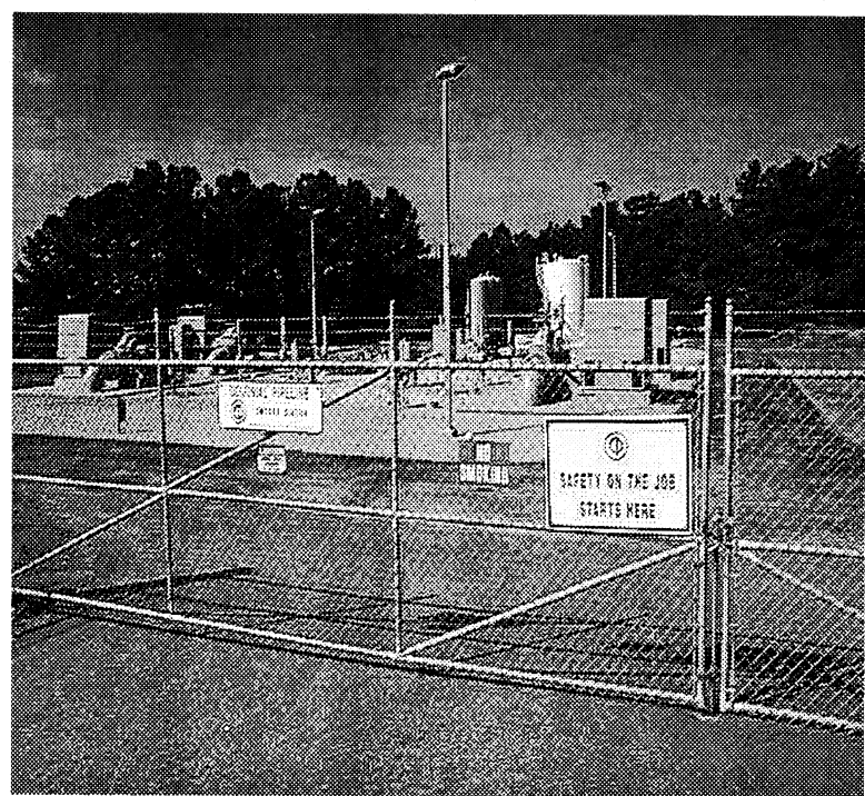
Four Westinghouse pumps help power over fifty thousand gallons per minute of gasoline and other distillates at Colonial Pipeline's Smyrna Pump Station, just 2000 feet from Cumberland Mall. Photo by Kea Vongchanh, Sting Staff
