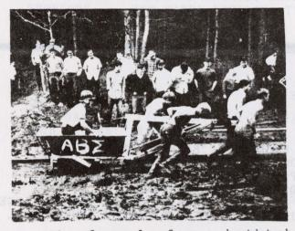
The formula for a bathtub racer is simple: take any cast iron, rolled rim bathtub four feet in length, acid-dip or grind it to the minimum 140 pounds, mount it on a lightweight frame, attach a 175 cc motorcycle engine, devise a steering system, install dependable brakes, and mount the whole thing on low profile Go-Kart racing slicks and you're in business.
