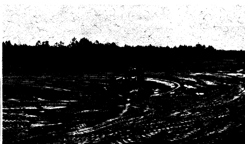
Leveling for construction of Norton Dormitory.
