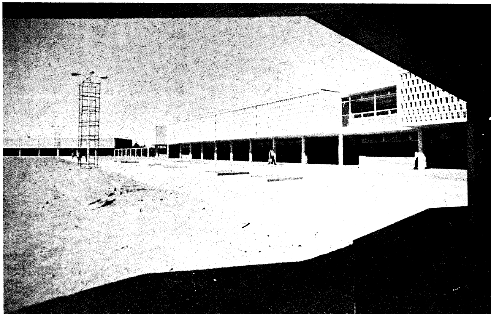
Completion of Classroom buildings at S. T. I.
